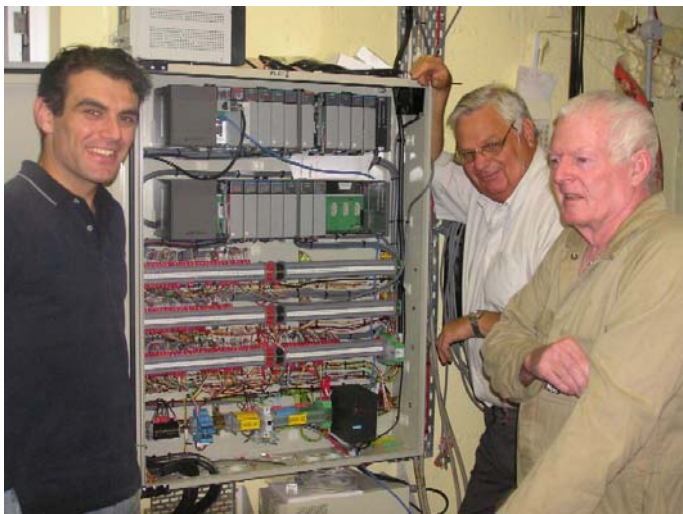
Figure 9: Con Costa, Clint Davies and Bob Ball at PLC2, controlling RF, ECH and Motor Generator
